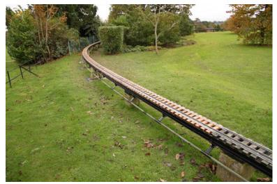
Rov P has led a team to replace a section of track from the jungle, partially up the straight towards the short tunnel. He has also scraped, wire brushed and repainted with bitumen about 75% of the steelwork around the track with a view to completing this task fully to give the whole ½ mile refreshed look and weather protection for
