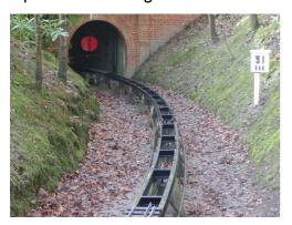
The track work is now complete with the final section ear-marked for repair between signal 4 and Wick Tunnel now complete, with re-painted steel work, 'turned' rail and re-treated sleepers. It was finally re-laid a couple of weeks back and all that remains will be a testing of the signals system in the early weeks of March in readiness for the new season on 25th. (See **Picture Left**).
